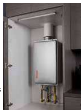
Example of an internal unit installed in a cupboard - Rinnai Auckland showroom
